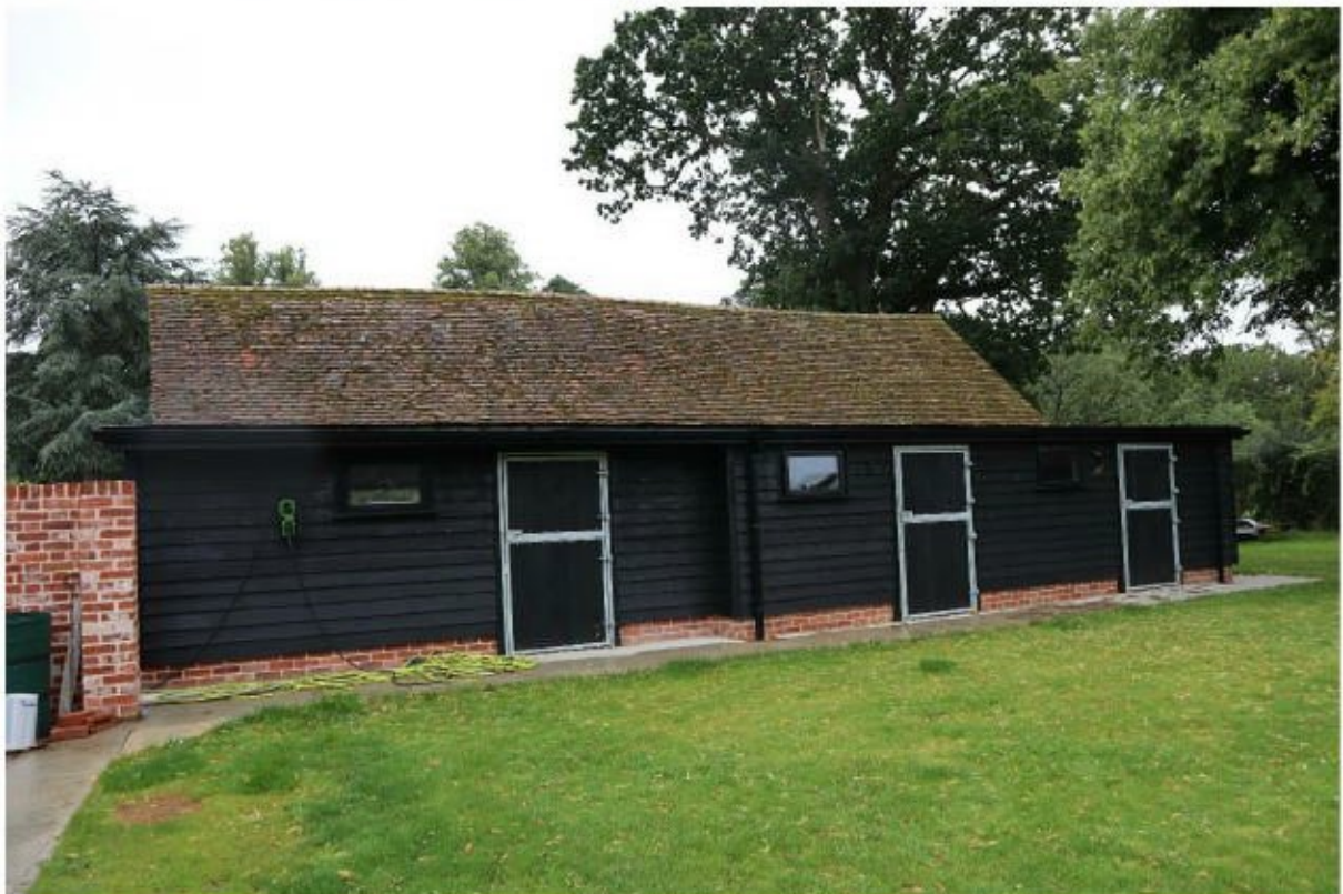
Figure 30 – rear of garage block.
