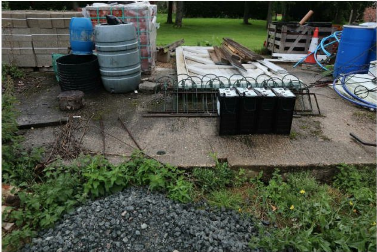
Figure 21 – concrete slab adjoining modern barn, to be used for extension.
