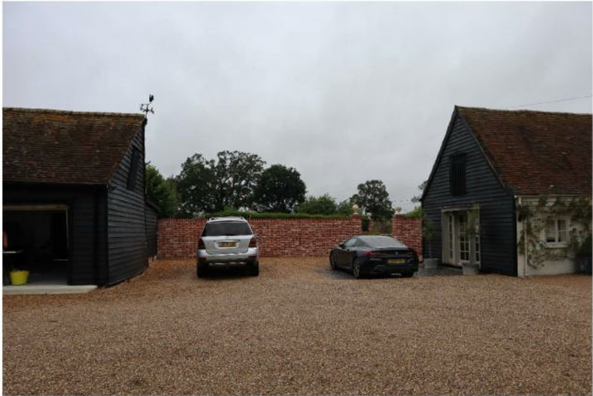
Figure 35 – garage block to the left, and the house to the left-hand-side, with the new wall screening view into the garden.
