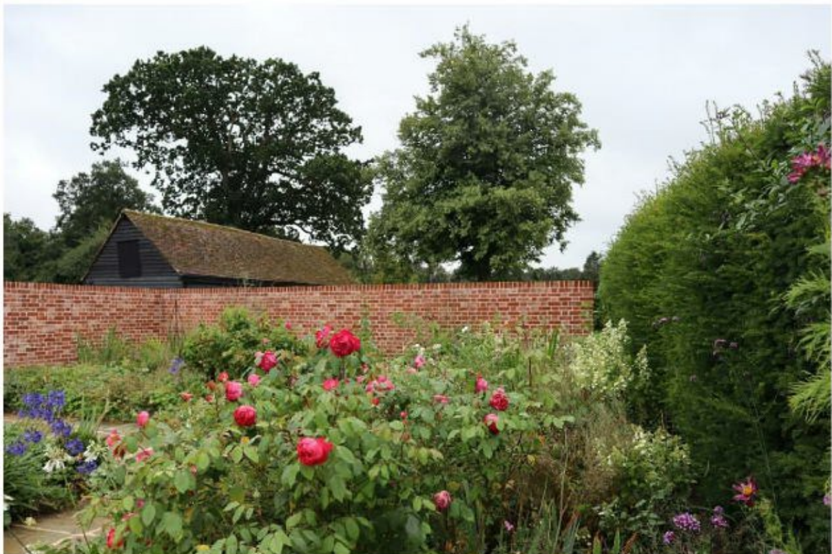
Figure 32 -looking from the Walled Garden towards the new wall and the rear of the garage block.
