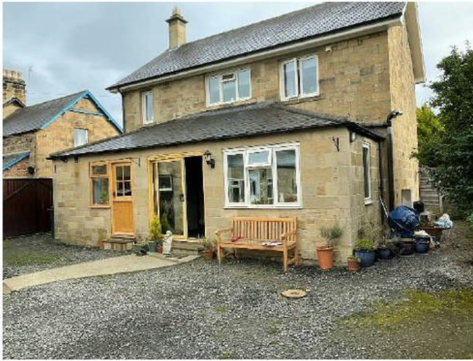
West facing Rear Elevation
