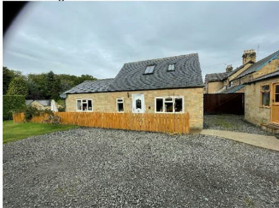
South Facing Elevation – Annex
