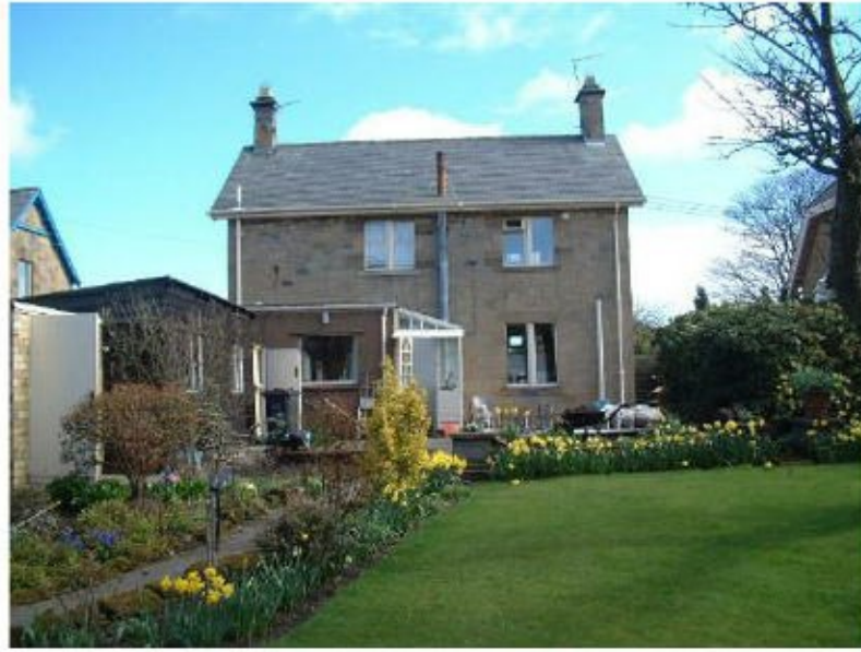
West facing Rear Elevation
