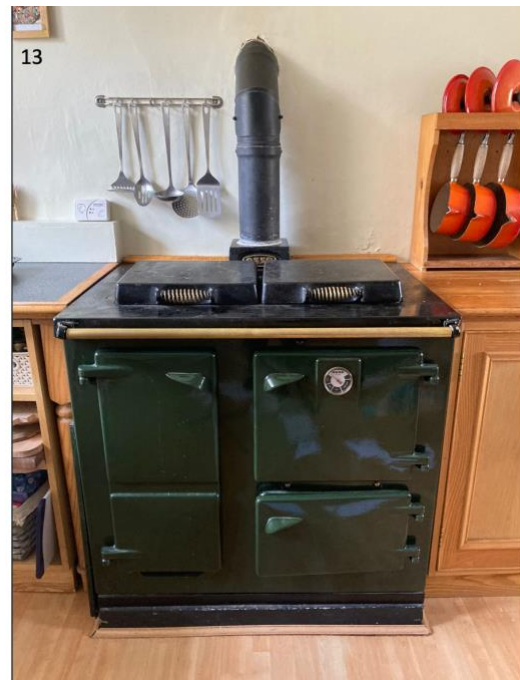
Figure 12: position and appearance of our Esse which is currently used for cooking and as a boiler for hot water generation and heating. We propose to remove it and to replace it with a modern but traditional looking electric range cooker.
