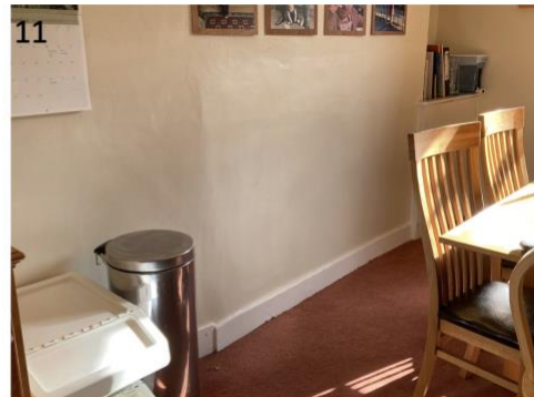
Figure 9: Positions of the new radiators we propose to install on the ground floor level. The radiator in the sitting room will go behind the sofa.
