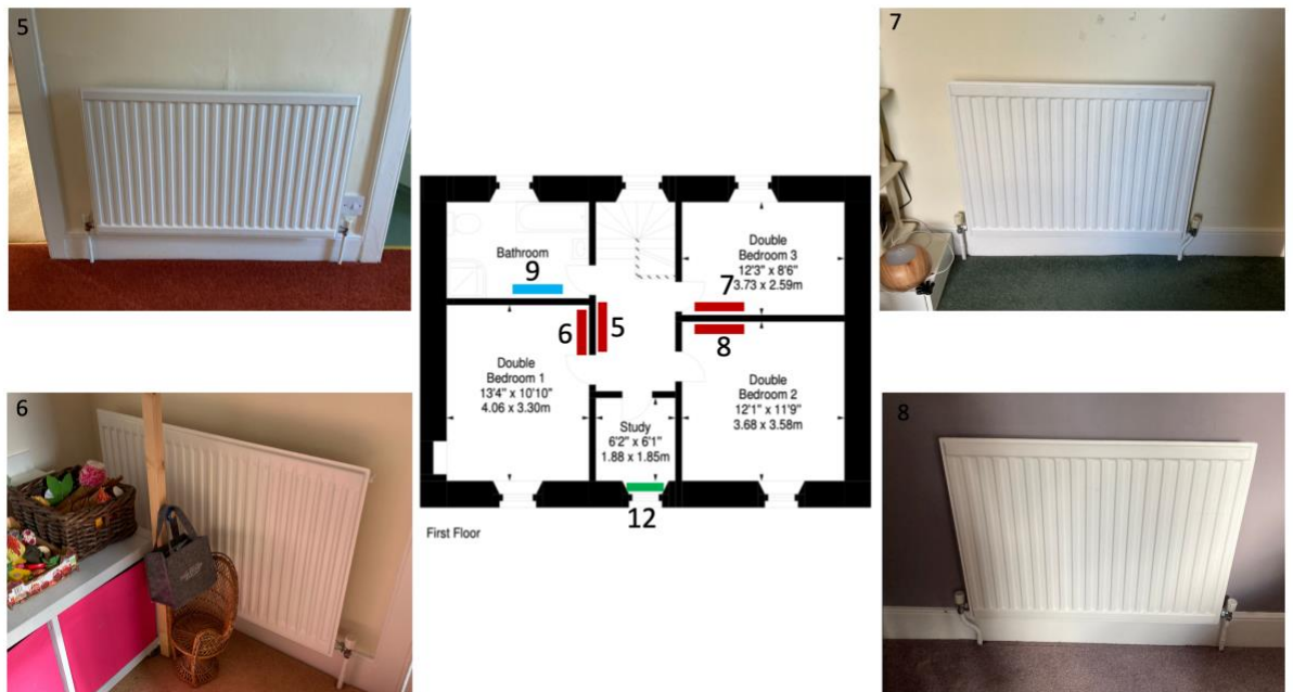
Figure 8: Photos of old radiators we propose to replace on the first floor. Their positions are marked on the floor plan in the middle.
