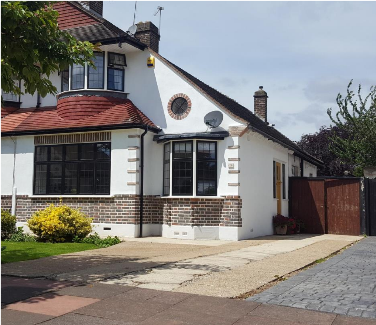
21 Frensham Road – front view from street
