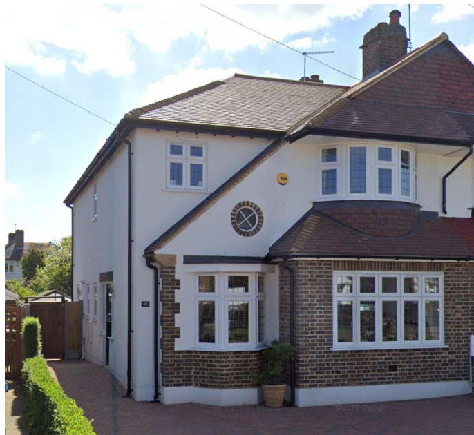
The design of the proposed extension reflects the appearance of 40 Telford Road (15/01226/FUL) and avoids an unsympathetic first floor overhang
