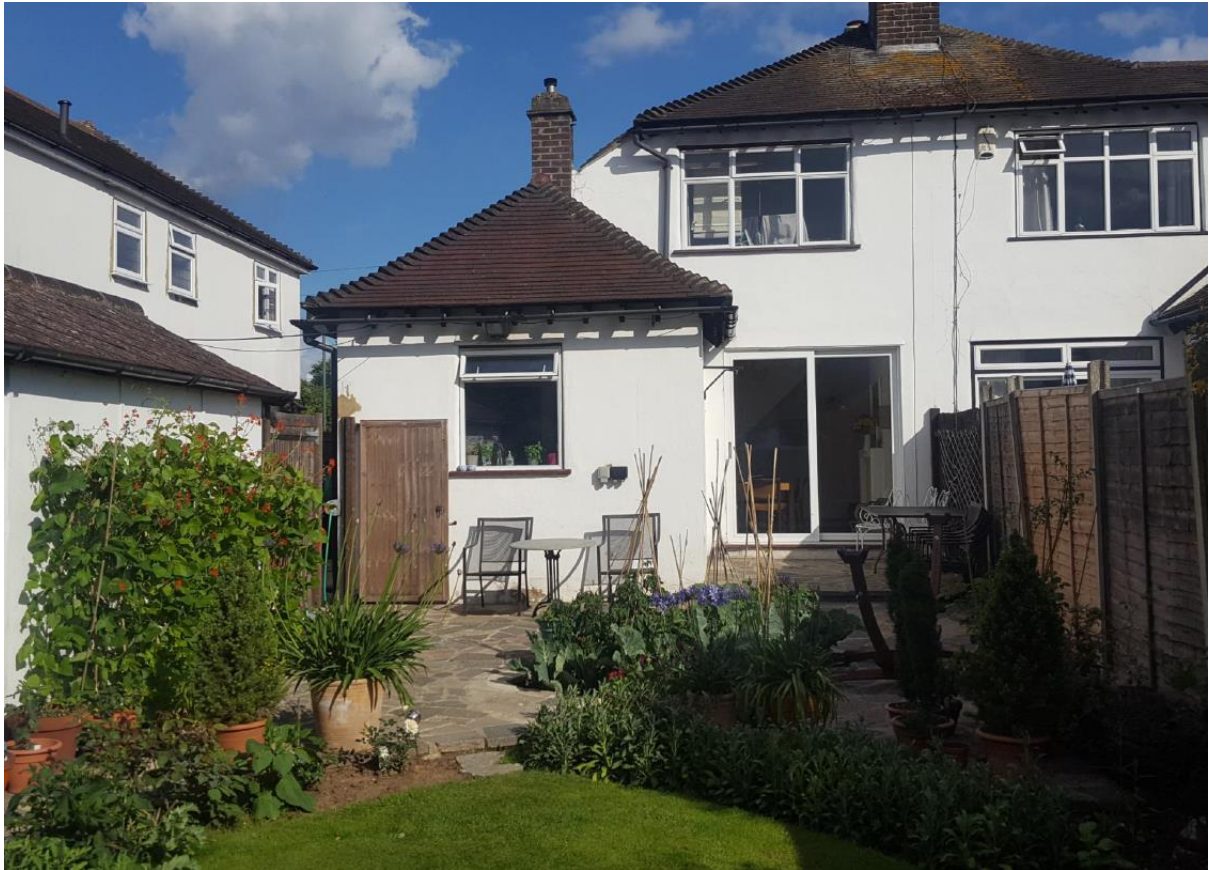
21 Frensham Road – rear elevation
