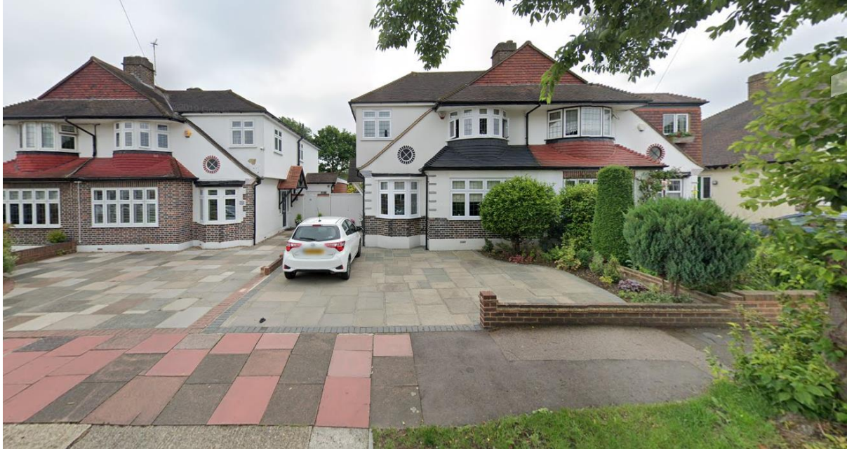
Nos. 24, 22 and 20 Frensham Road have all been subject to first floor side extensions with hipped roof forms
