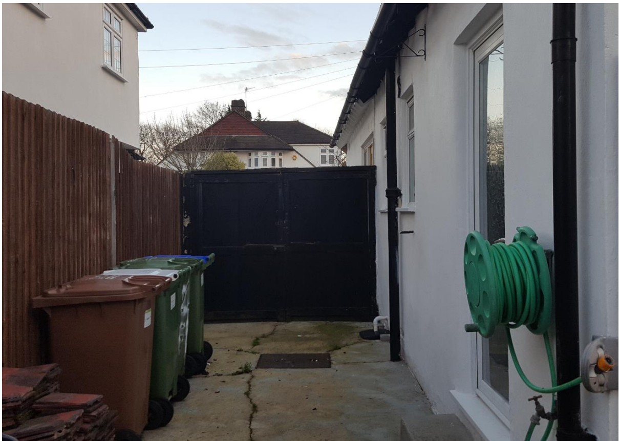
21 Frensham Road – side driveway
