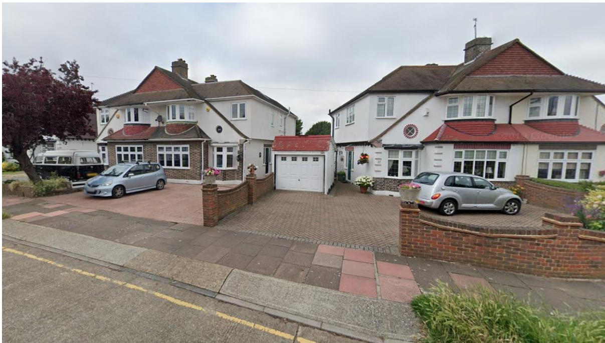
Nos. 23, 25 and 27 Frensham Road have also all been subject to first floor side extensions with hipped roof forms
