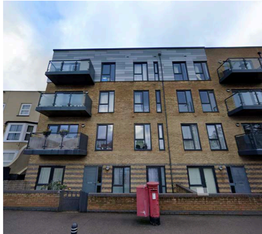
1. Modern apartment block on Watling Street
