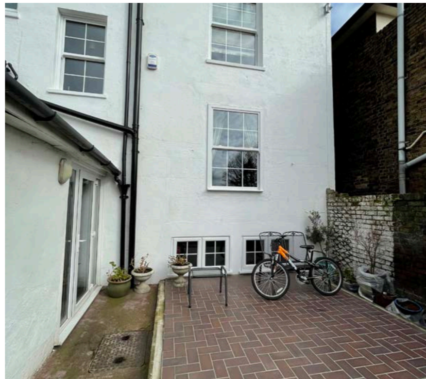
3. View from the garden towards the east boundary
