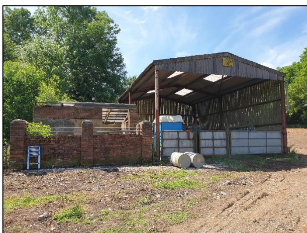
Building B1 – view looking south
