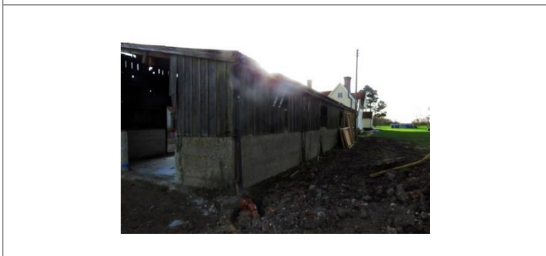
External view of the old cattle shed External view of the old cattle shed
