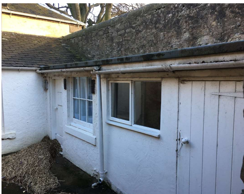
Below: Kitchen and utility within the West courtyard
