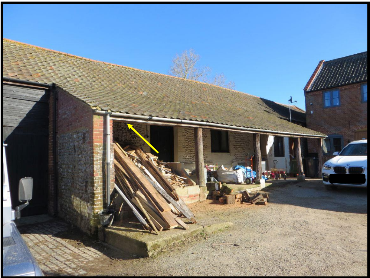
Plate 5: Emergence point (southern elevation) where main external wall meets shelter
