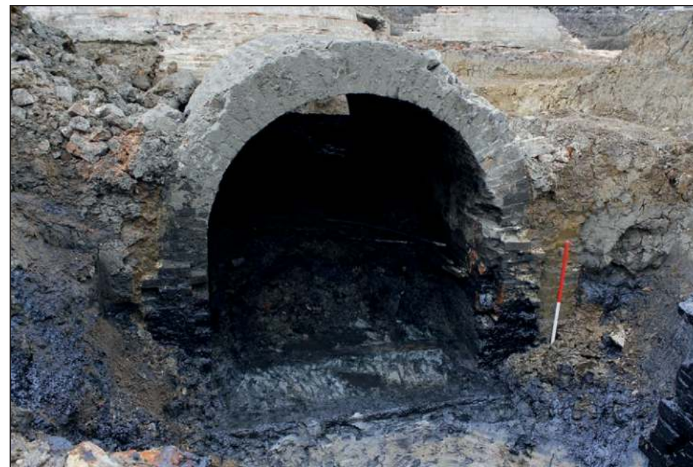
Culvert 1520, looking north (1m scale)
