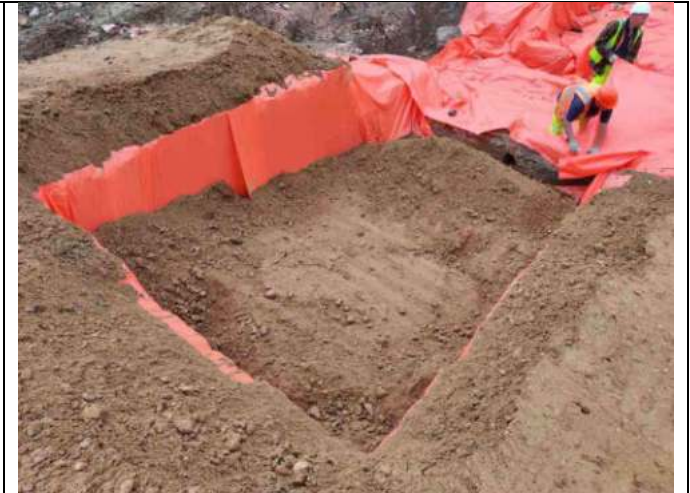
Central archaeology, installation of terram and 300mm sand 23/09/2020
