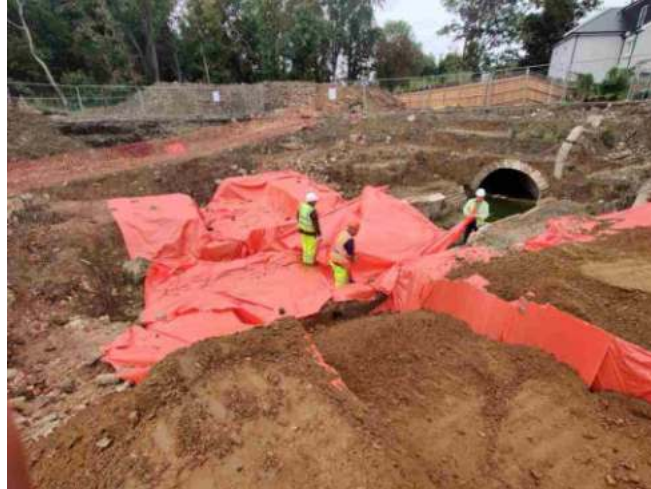
Central archaeology/culvert, installation of terram and 300mm sand 23/09/2020
