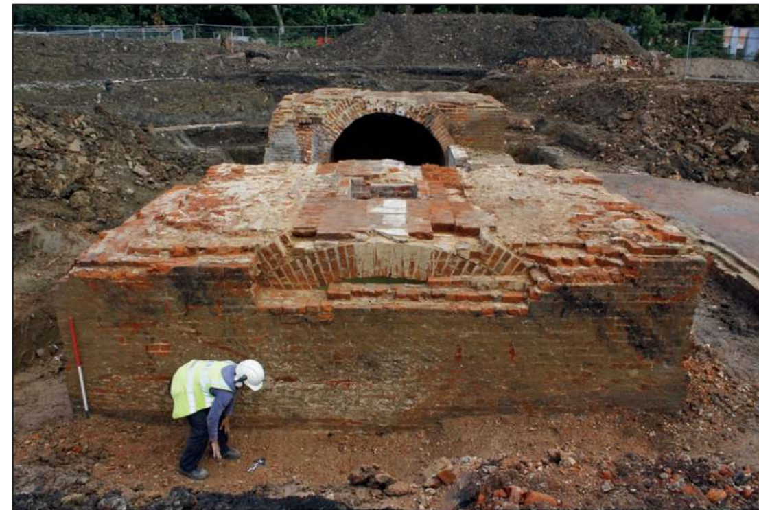
View north-west towards South Vault 1.2 (Powder Mill A), (Period 2). Blast Wall 1.9 (Period 2) and later Corn Mill remains (Period 3) have been removed
