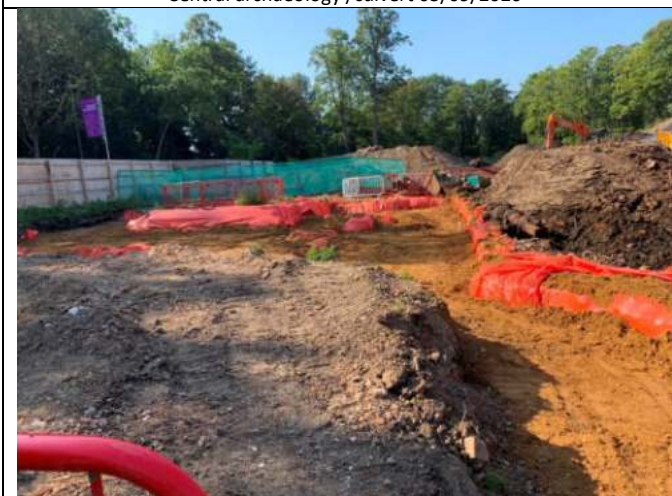
North archaeology, installation of terram and 300mm sand 21/09/2020
