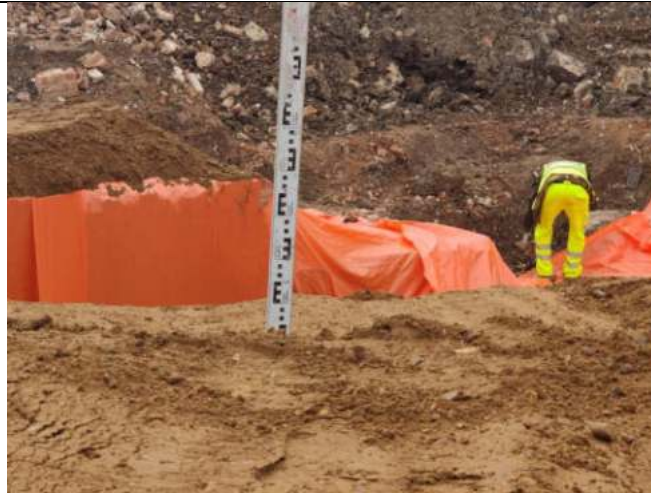
Central archaeology, installation of terram and 300mm sand 23/09/2020
