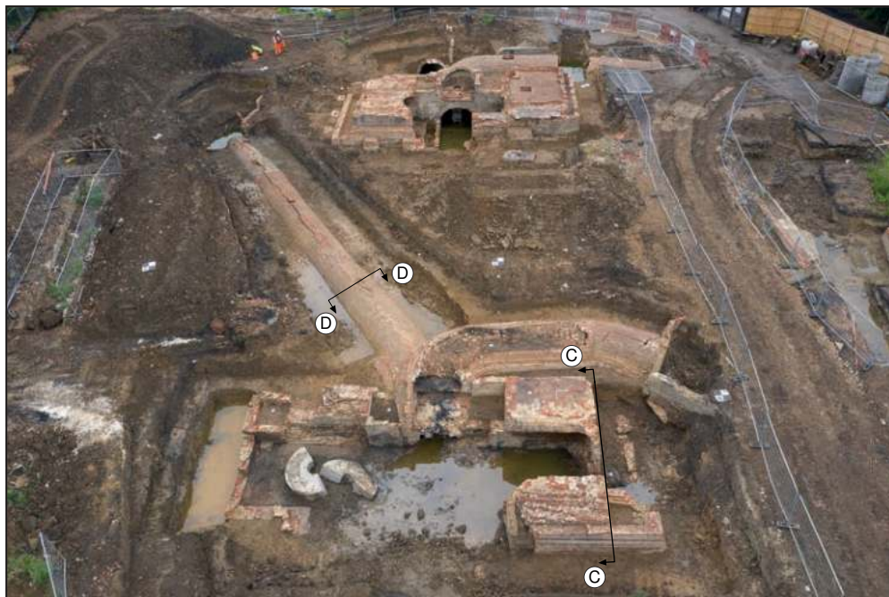
Powder Mill B (view north-east)
