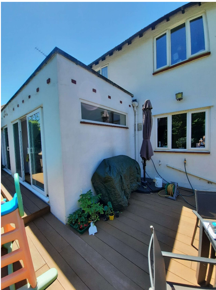
Side of rear extension
