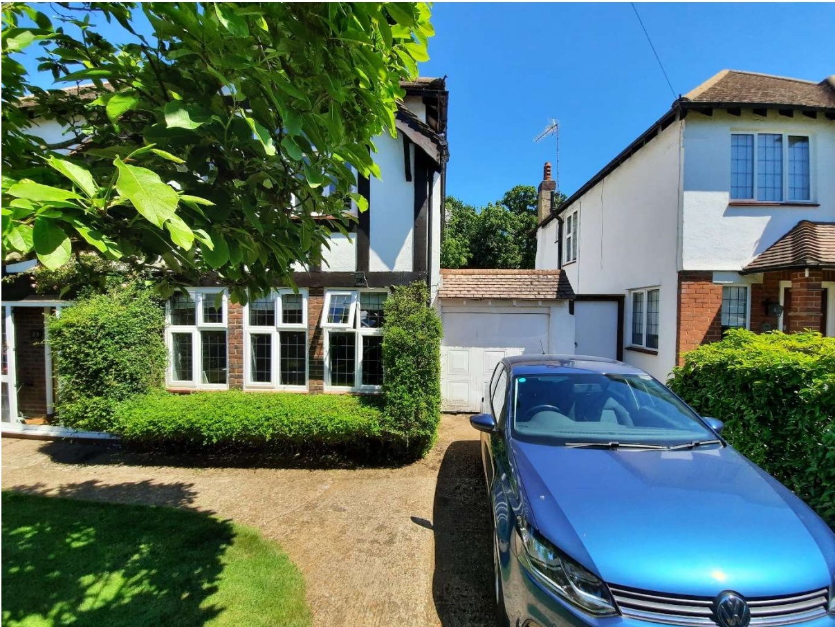
Front elevation showing garage and no.81
