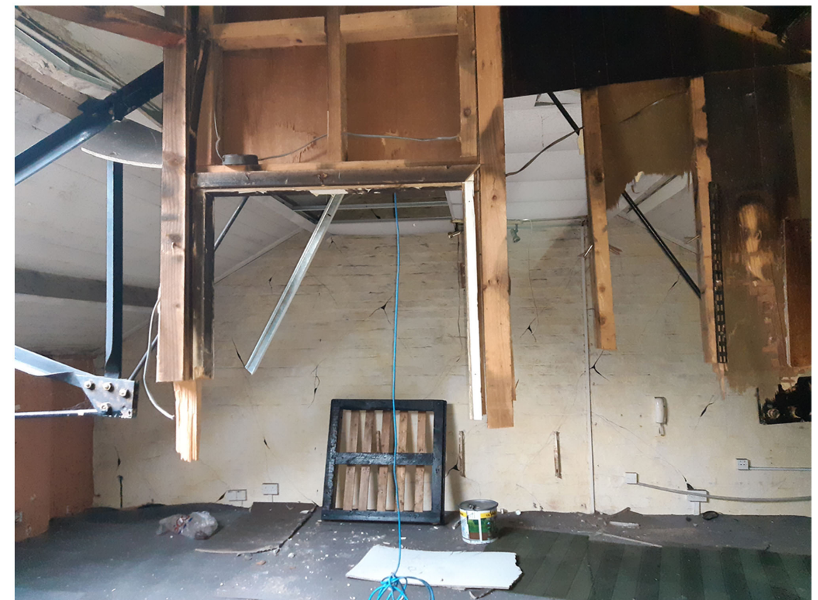
Above: condition of existing mezzanine and roof
