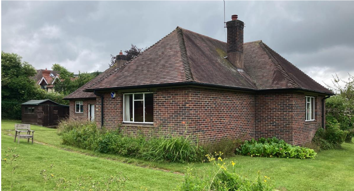
Fig 3 View looking towards the rear of the existing property
