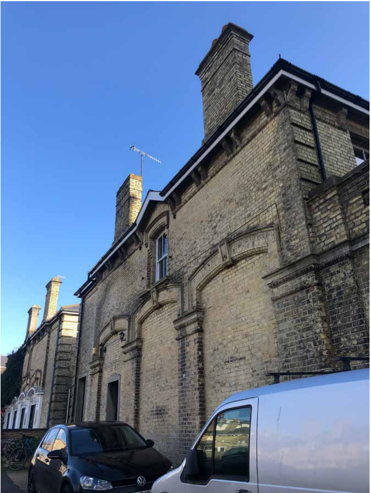
26. The side (west) elevation of 56 First Avenue, February 2020 (Donald Insall Associates)
