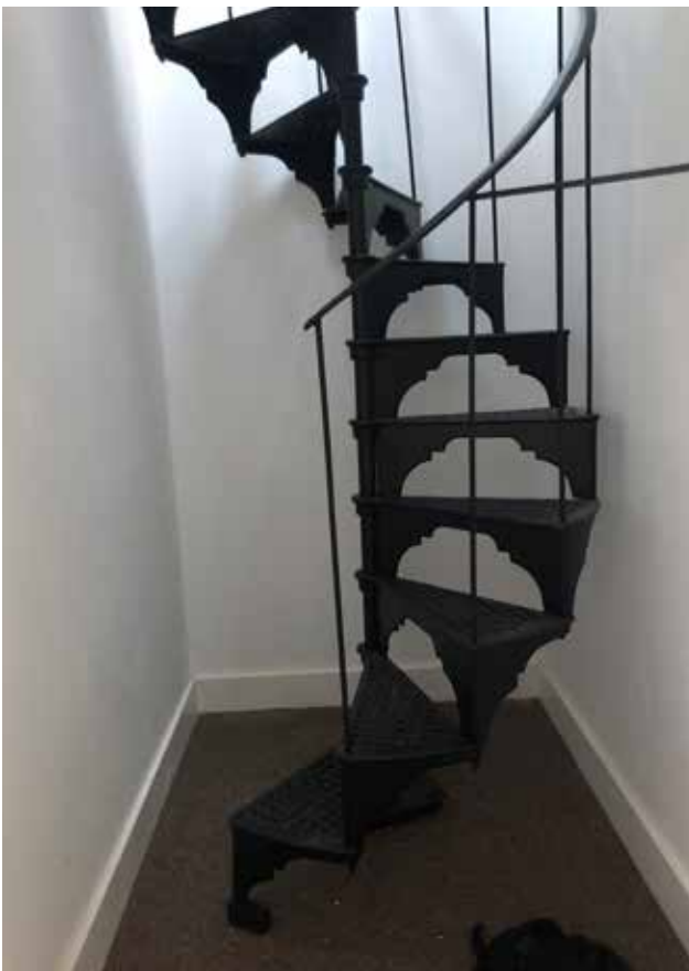
35. The unconsented relocation of the late-20 th century spiral staircase in room F4, February 2020 (Donald Insall Associates)
