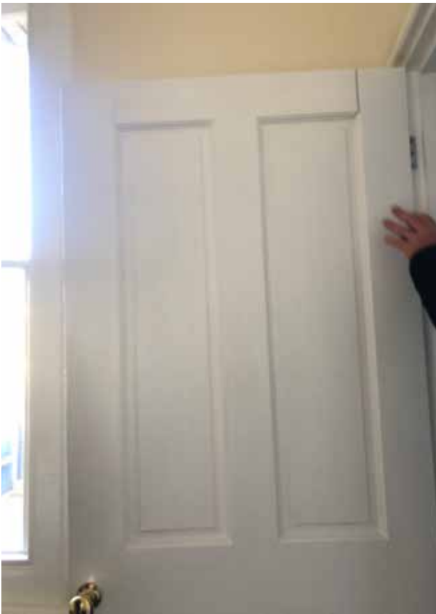
29. The modern four-panel door to room F2, February 2020 (Donald Insall Associates)
