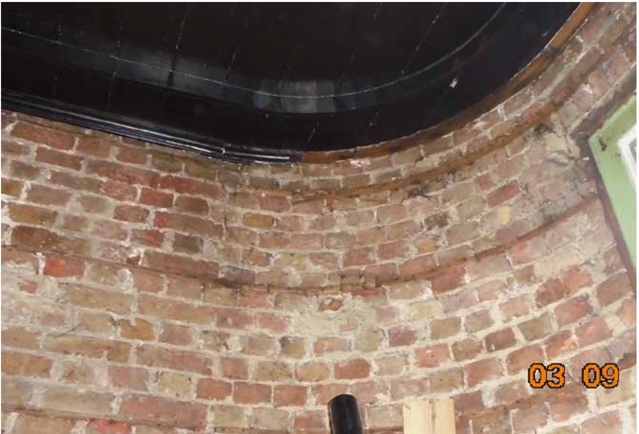
27. Brick interior of room G2, September 2019 (Brighton and Hove Planning Archive)
