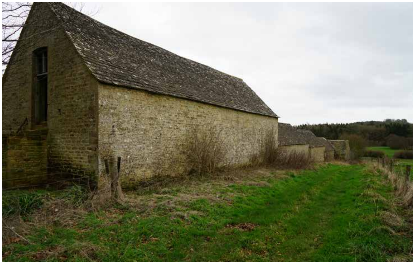
The north and western side wall with the buildings to the southern end stepping down the slope
