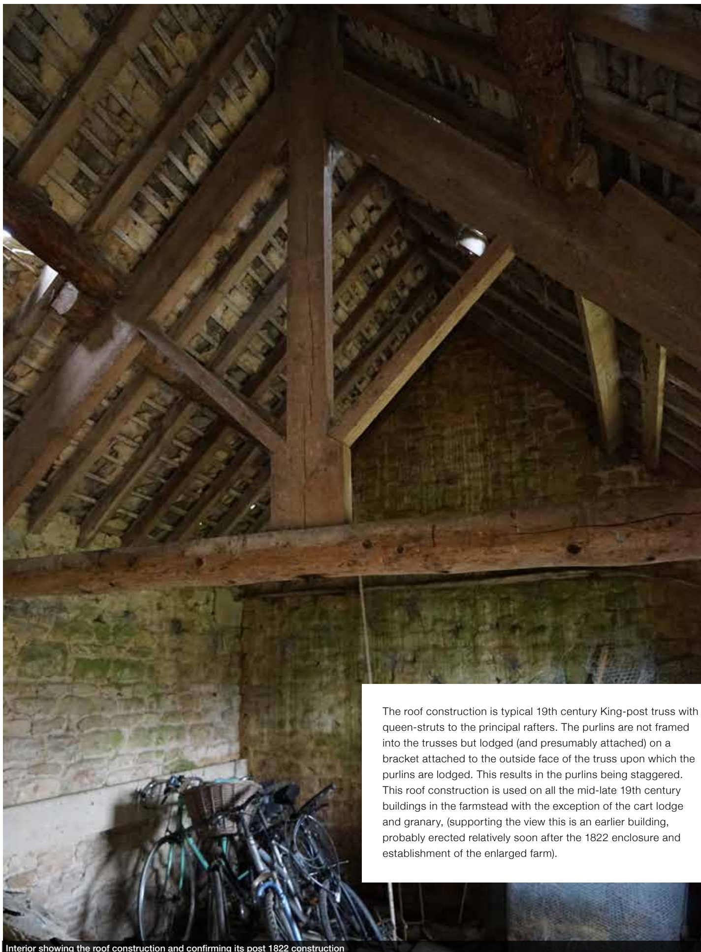
Interior showing the roof construction and confirming its post 1822 construction
