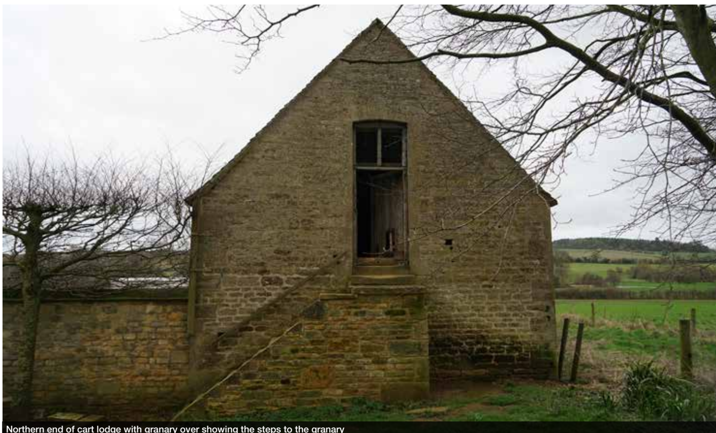
Northern end of cart lodge with granary over showing the steps to the granary
