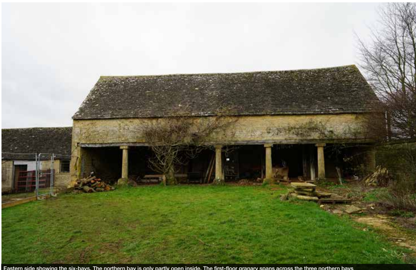
Eastern side showing the six-bays. The northern bay is only partly open inside. The first-floor granary spans across the three northern bays
