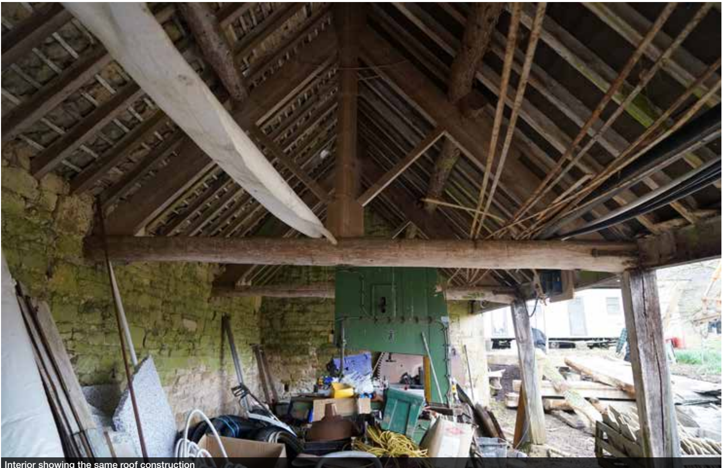
Interior showing the same roof construction
