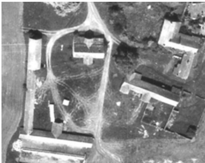
Aerial image showing the farmstead layout. Note the yard between the Standing Barn and the cart lodge and granary is open providing evidence that the current walled enclosure post-dated 1975. There is a low wall enclosing a yard to the rear of the south range
