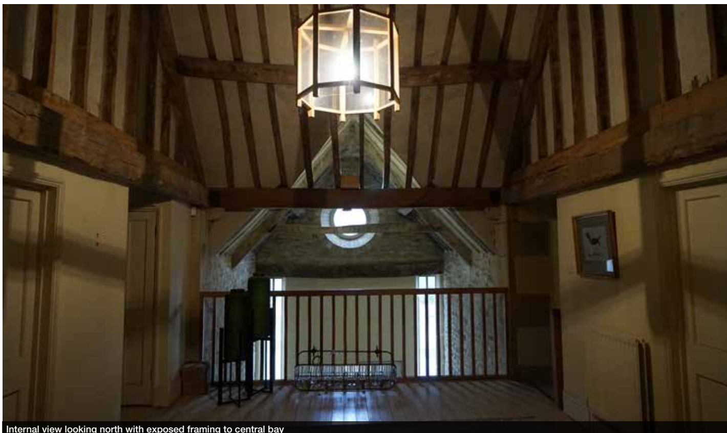
Internal view looking north with exposed framing to central bay
