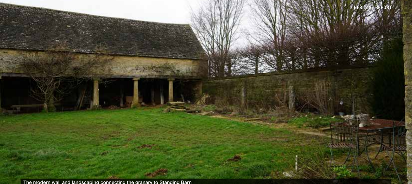
The modern wall and landscaping connecting the granary to Standing Barn
