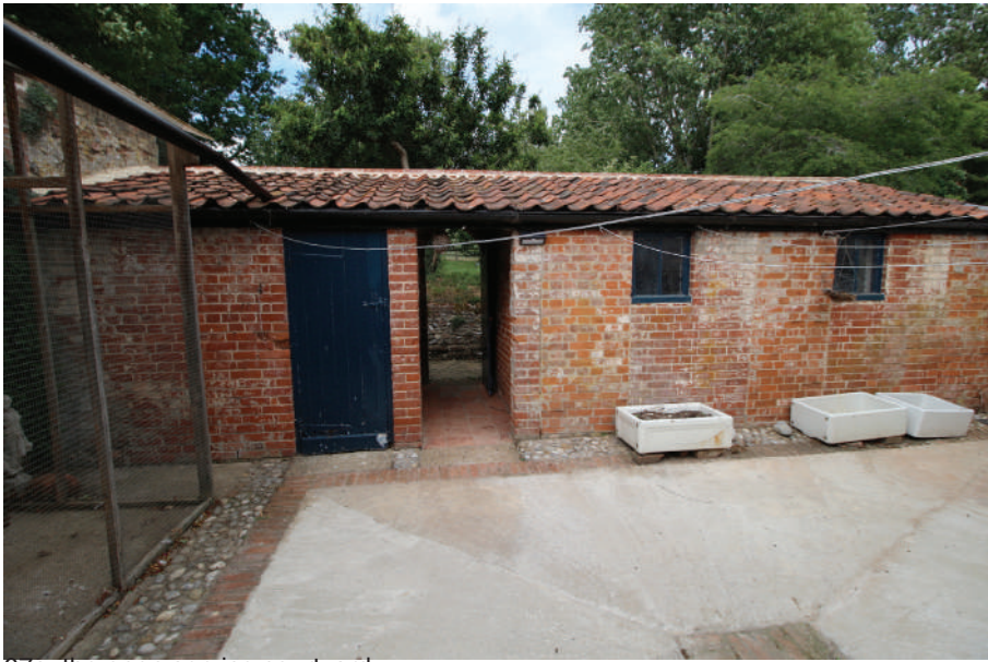
07a: the open service courtyard
