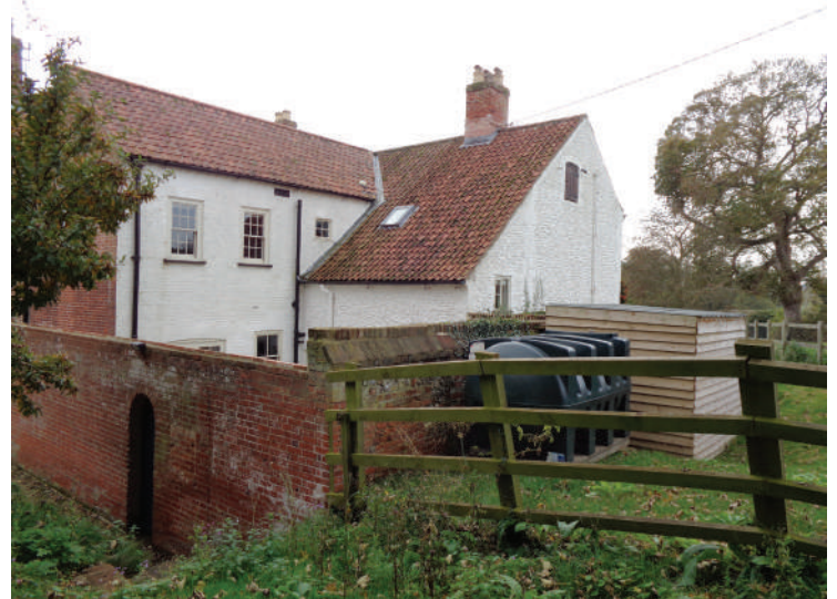
12: View from the north (churchyard and public footpath), the fence will be replaced by hedging and the oil tank & water treatment plant relocated
