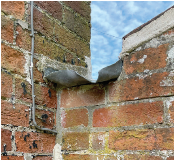
13: the roof level junction between the outbuilding and house
