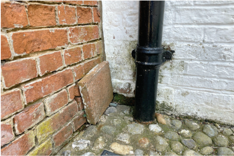
09: The rainwater pipe that serves the main house and outbuilding
