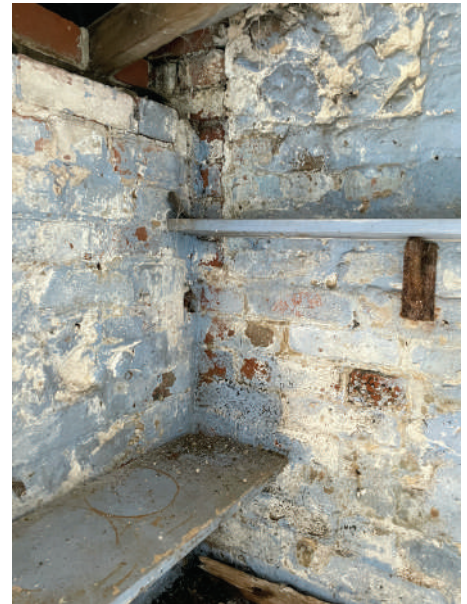
08: the internal face of the external walls of the outbuilding
