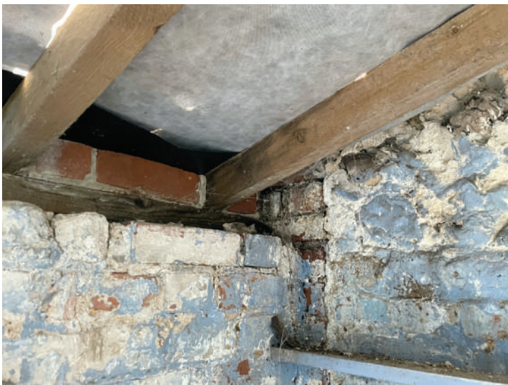
11: Modern rafters to the monopitch outbuilding
