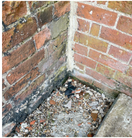
14: Floor level junction between house & outbuilding
