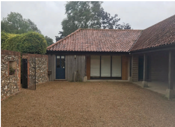
15: The annexe is a modern stand alone building comprising a accommodation on 2 floors and an open cartshed. The cartshed will be partially enclosed to provide a plant room to serve the gym & house
