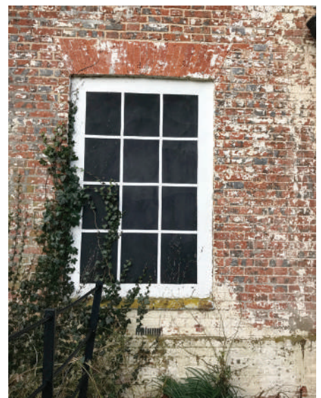
06: a blocked ground floor window
