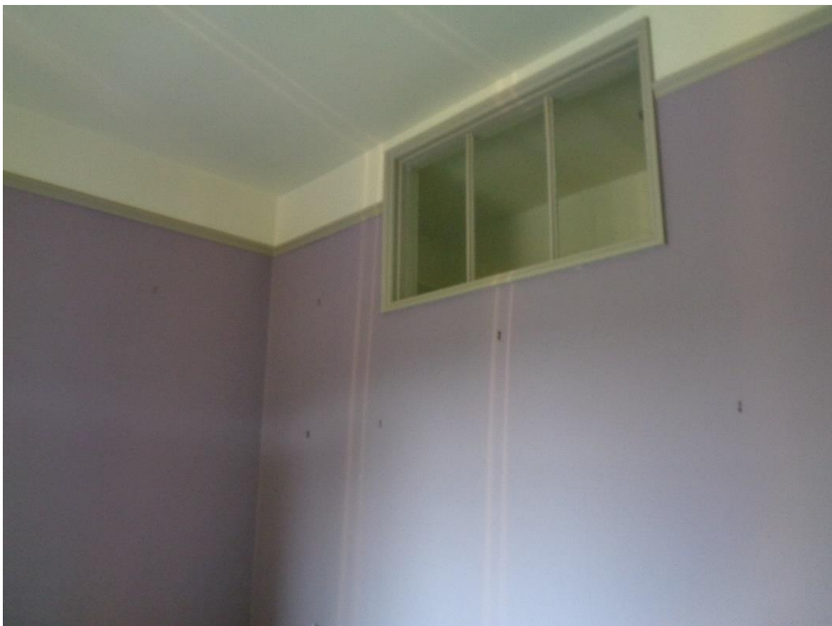
Internal window lighting corridor
