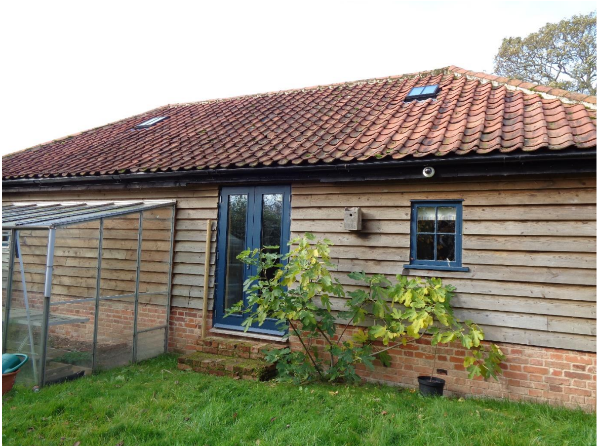
Detached outbuilding adjacent to lane
