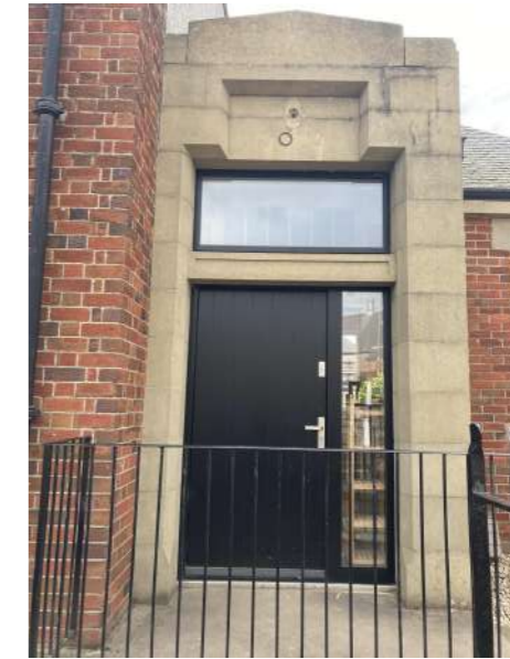
Northeast front door entrance
