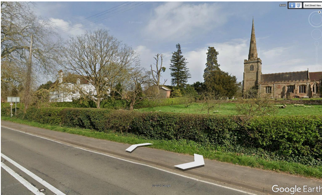
Figure 6 – View from A448 showing church of St Cassian with adjacent modern barn (to centre of photo)
