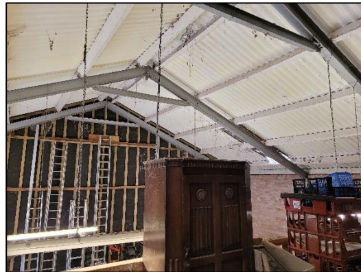
Plate 4: Showing a view of the roof structure inside the barn.
