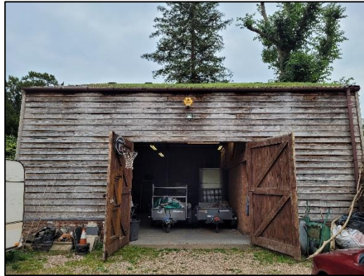
Plate 1: Showing a typical view of the barn. Photograph looking east.
