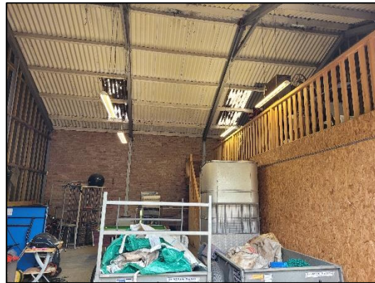
Plate 3: Showing a typical internal view of the barn. Photograph looking west.
