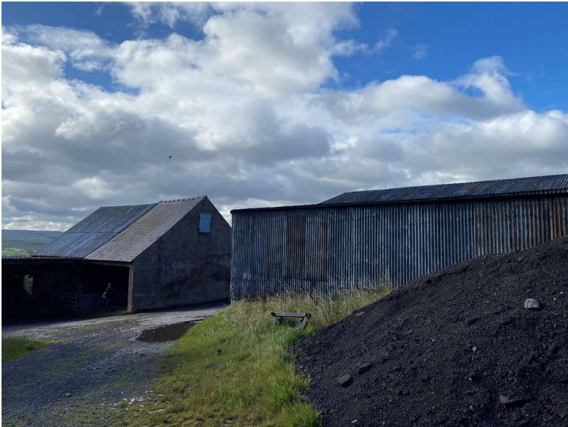
View of existing buildings
