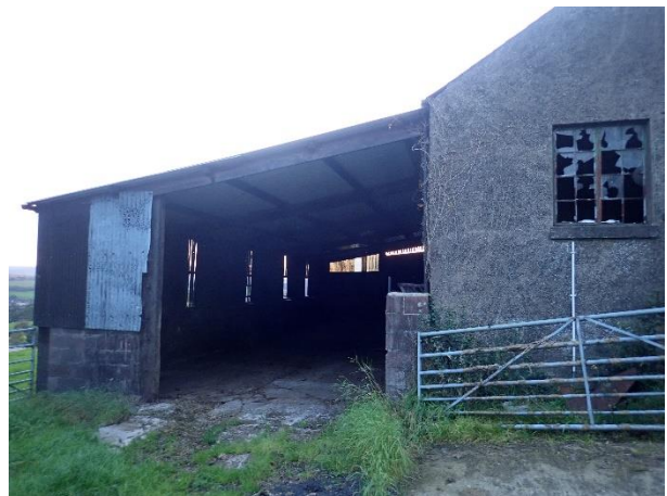
Building A and B from the southwest
