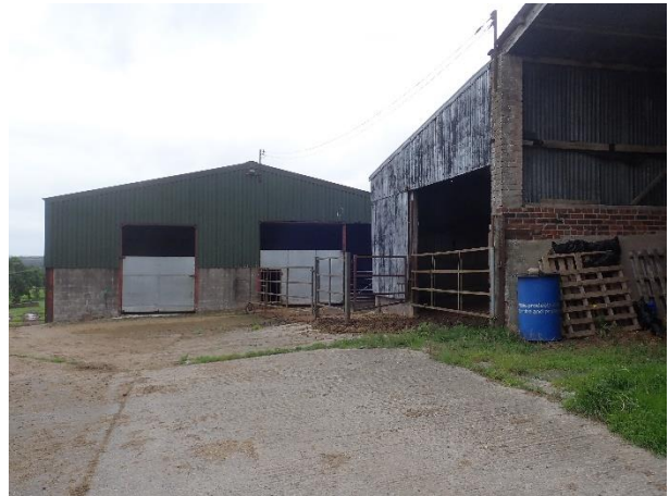
Building G (and F) from the east
