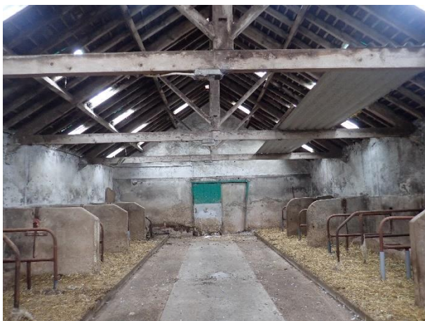
Interior of Building A
