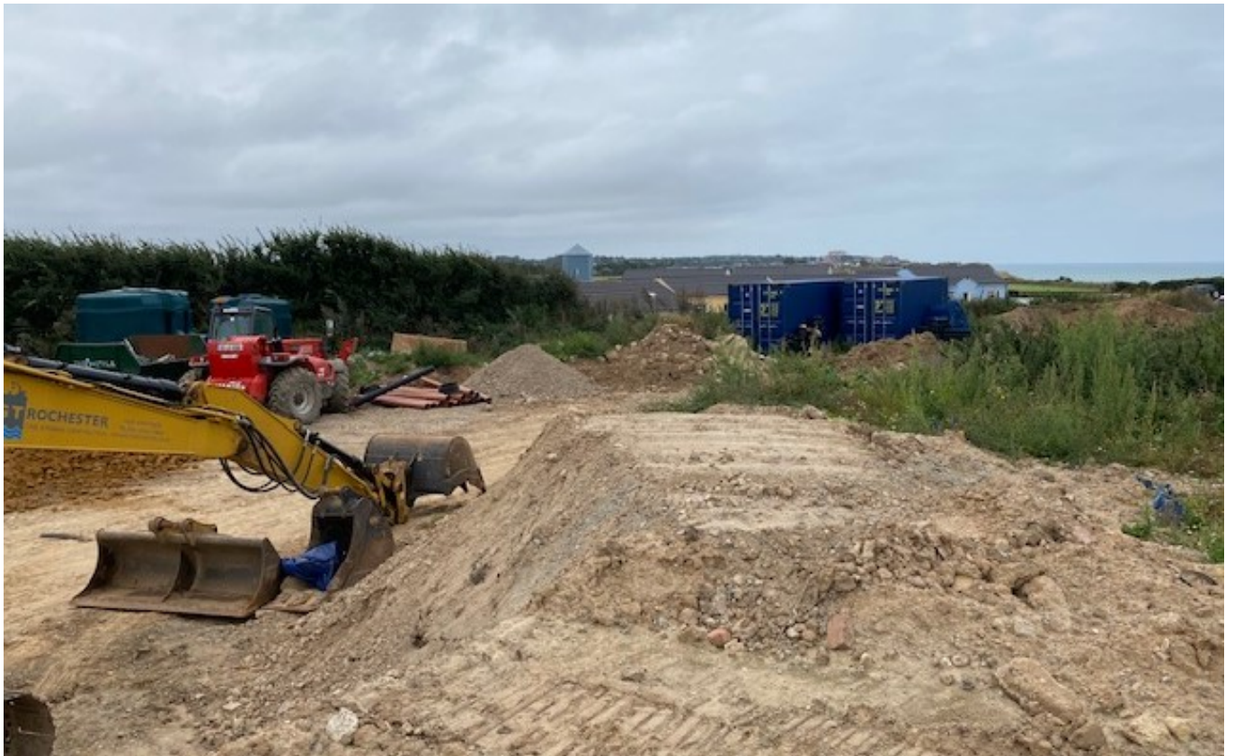
Plant and materials storage.
