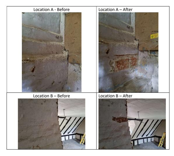
Existing masonry paint will only be removed from external render where it has become loose and detached from the render. No chemicals or manual scraping will be used to avoid damaging the existing lime render. The Pozilime limewash which will be used to paint is a breathable limewash that can cover different surfaces so can be overpainted on to the existing areas of lime, concrete and areas of remaining masonry paint.
