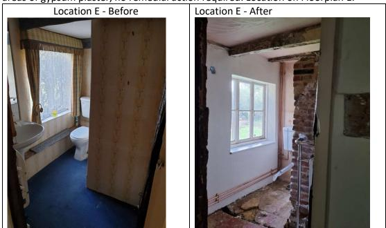
Photo showing Downstairs Bathroom/Service end before with fibreboards lining the walls and subsequent photo of exposed walls with fibreboards removed. No damage to underlying fabric, walls in good condition, composed of lime and no remedial action required. Location on Floorplan F.
