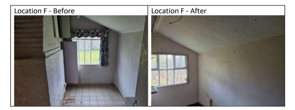
Photos showing areas of concrete render to be removed and photos of render removed. Location on Floorplan G, H and I. Most existing Riven Chestnut laths in good condition, brickwork plinth in good condition.
