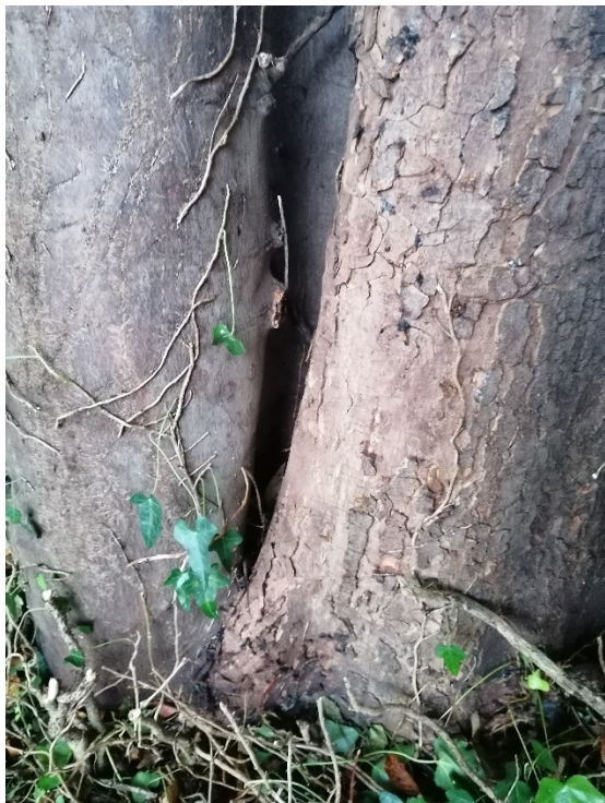
Picture 2. Tight union at base of tree with rainwater cavity forming.
