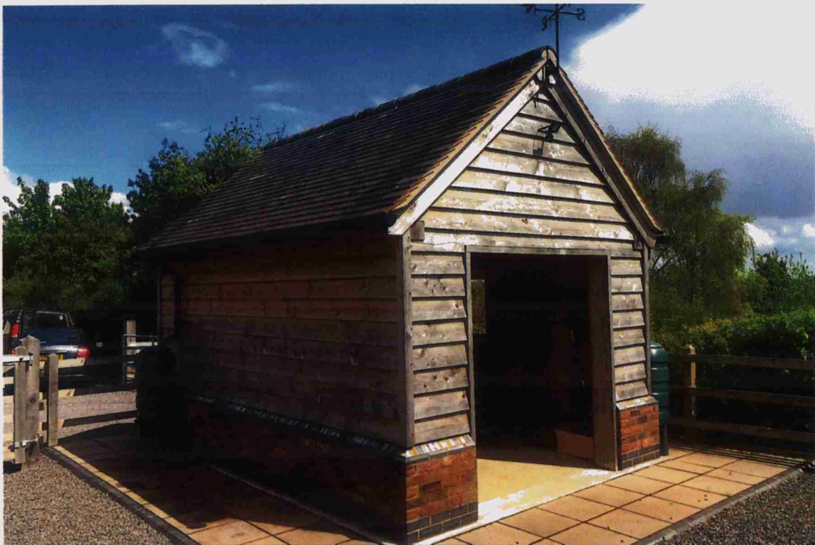
PHOTOGRAPH 5 - DETAIL OF THE IMPLEMENT STORE WHICH WAS CONSTRUCTED AT BIRCHFIELD COPPICE. THE PROPOSED BARN WOULD USE SIMILAR MATERIALS.
