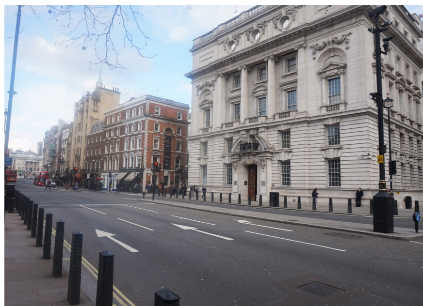
View looking north along Whitehall
