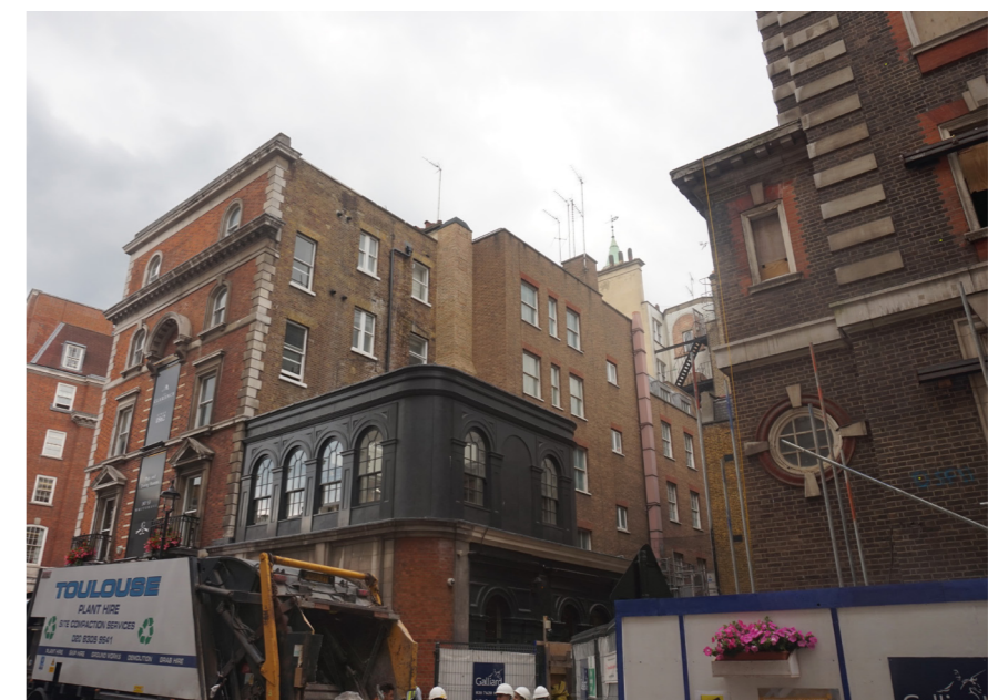
Rear of site viewed from Great Scotland Yard
