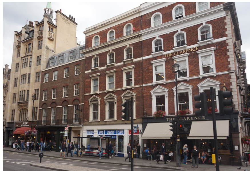
Existing shopfront is a poor relation to its neighbours either side
