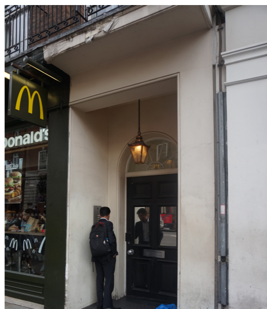
The existing office entrance is narrow and cramped
