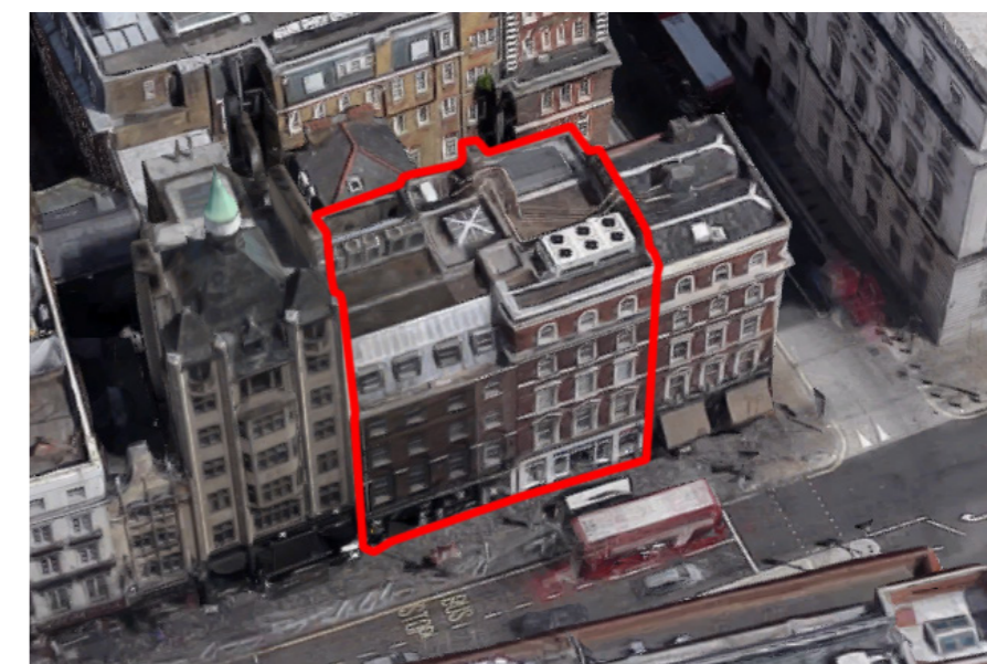
Aerial view from the west
