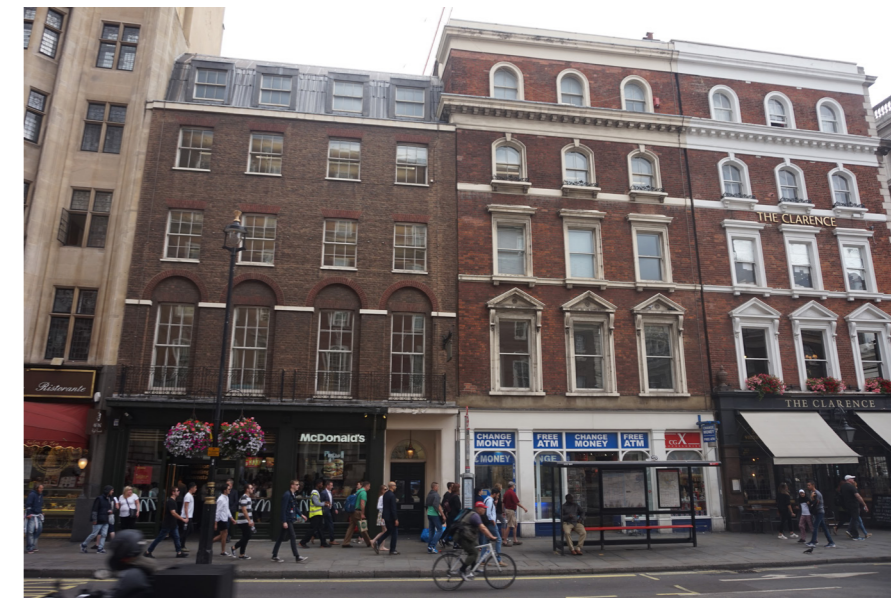
View of front facade
