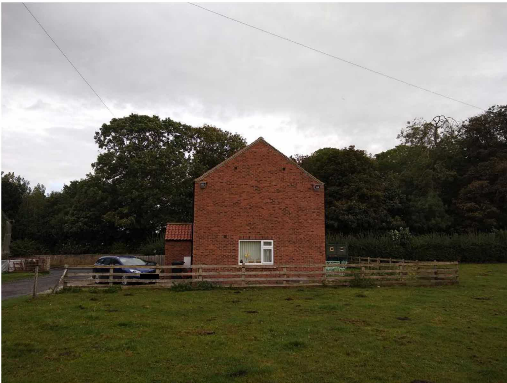
2. Photo of existing boundary fence to the side of the property.
