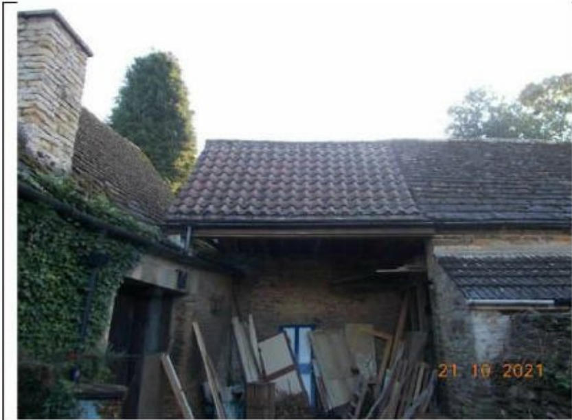
Plate 6: Building 2. Photograph taken from the west.
