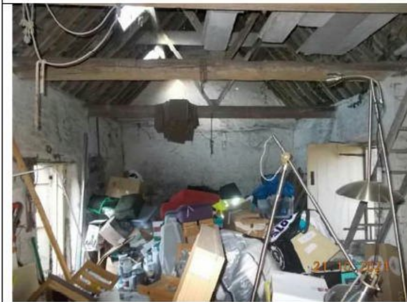
Plate 2: Building 1, showing the room at the western gable end.
