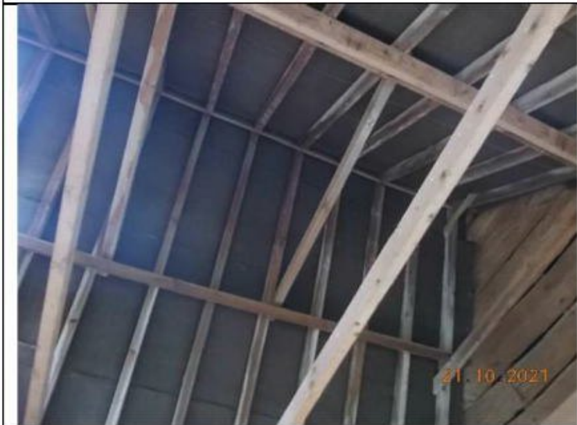
Plate 7: Building 2, showing the lined roof.
