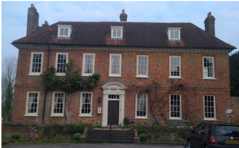
Fig 3 The Old Rectory, front elevation
