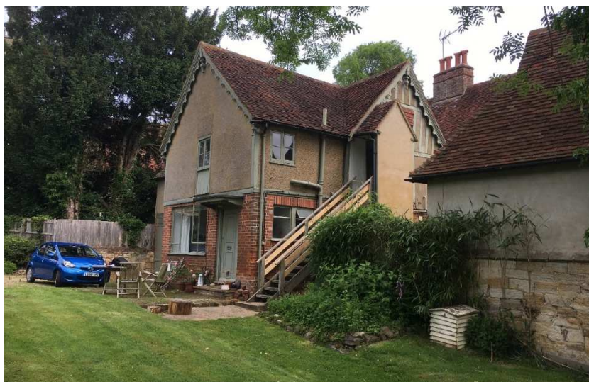
Fig 4 Former stable and coach house
