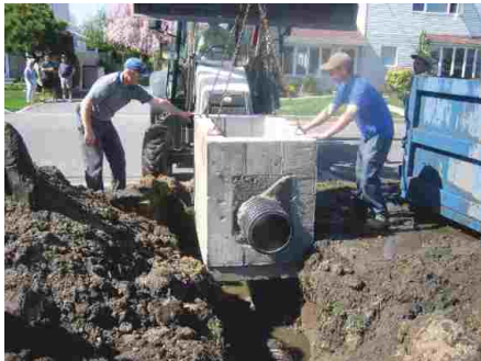
Smaller Smart Filter ® being lowered into position
