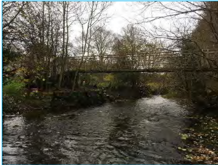
Figure 3 - Footbridge Adjacent to the Site Looking Downstream
