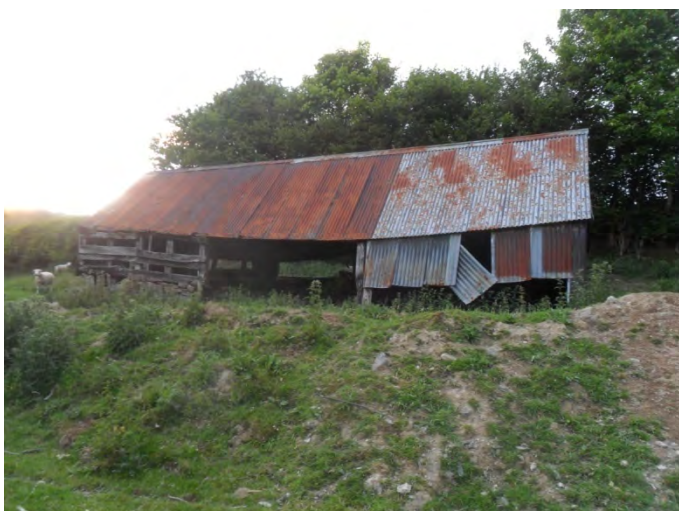
Missing/displaced tin sheeting, open front, ridge capping
