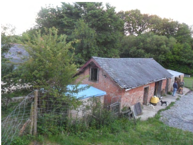
Open windows/doorways, missing slates, under ridge
