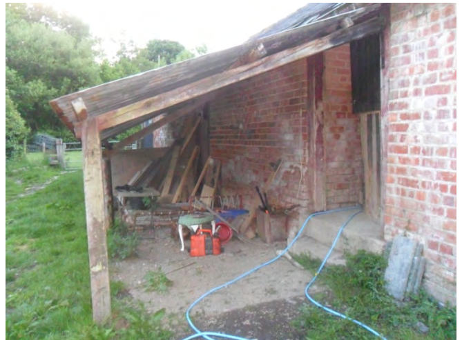
Lean-to at eastern aspect
