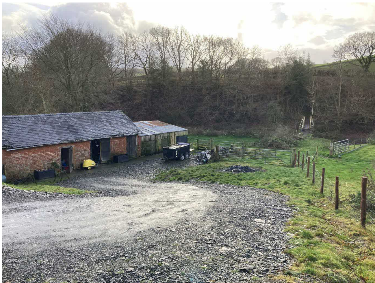
Photograph 3: Southern part of the site looking S
