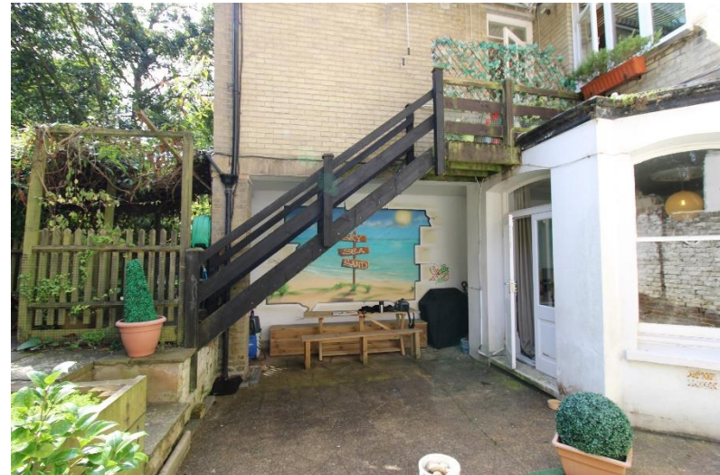
Photo from Garden looking toward undercroft area.
