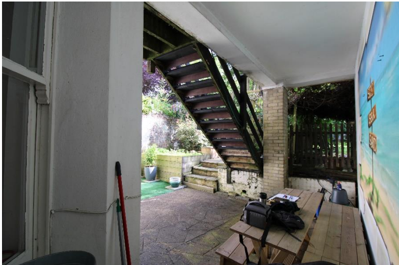
Photo from undercroft area facing toward garden.
