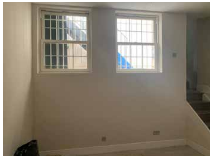
Photo 6 - Lower cellar area
