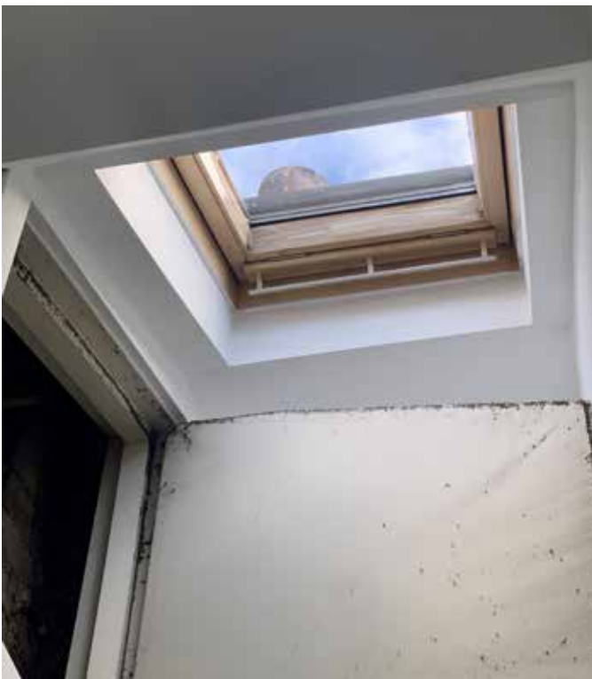
Photo 15 - Existing rooflight over family bathroom on second floor
