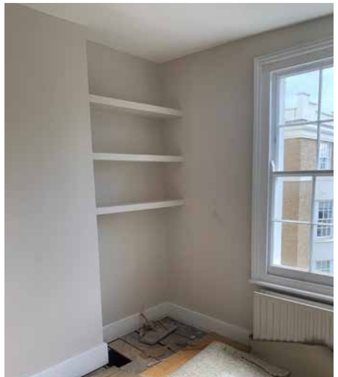
Photo 16 - Existing second floor rear bedroom
