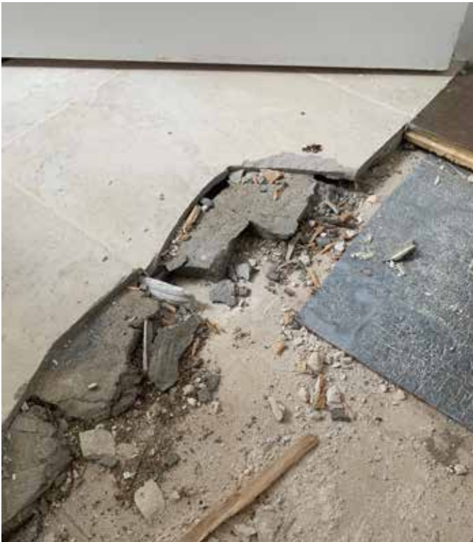
Photo 3 - Existing screed uncovered to Basement
