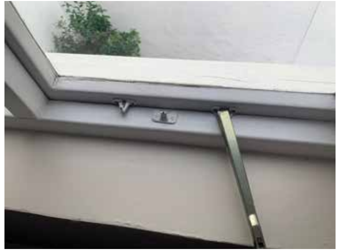
Photo 8 - Existing window in ground floor rear room
