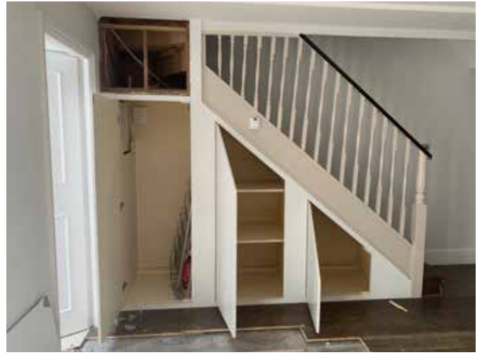
Photo 2 - Existing ground floor to Basement stairs
