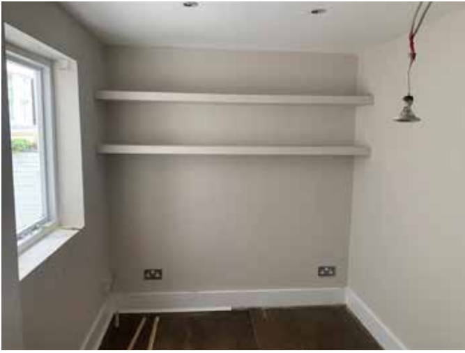
Photo 7 - Existing ground floor rear room
