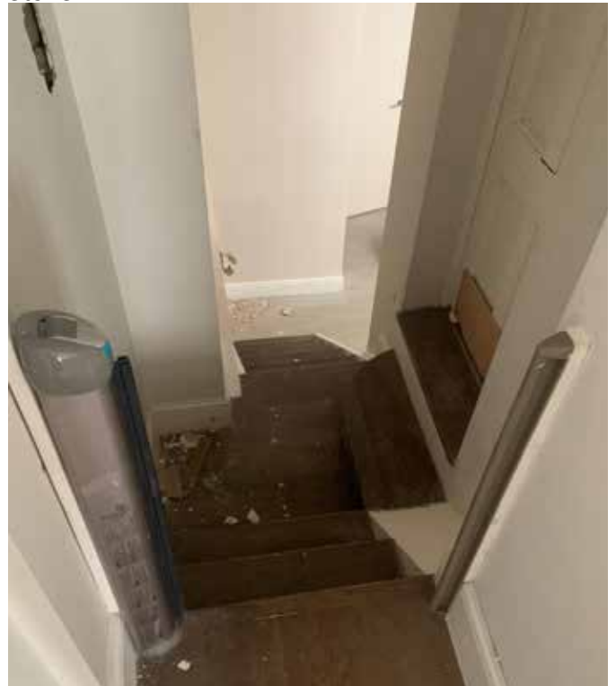
Photo 4 - Existing stairs down to lower cellar area
