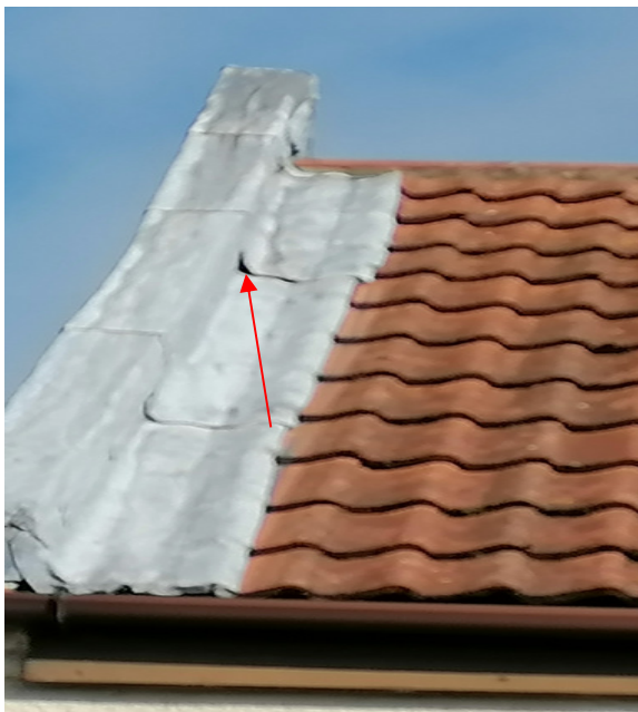
Plates 10 & 11. Shows lifted flashing and east gable
