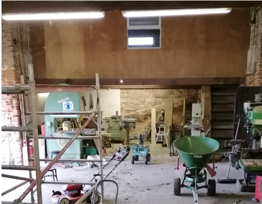
Plate 18. Shows boarded room to east gable.
