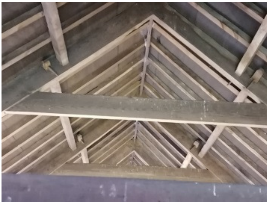
Plate 19. Shows timber roof trusses and bit mastic felt lining.
