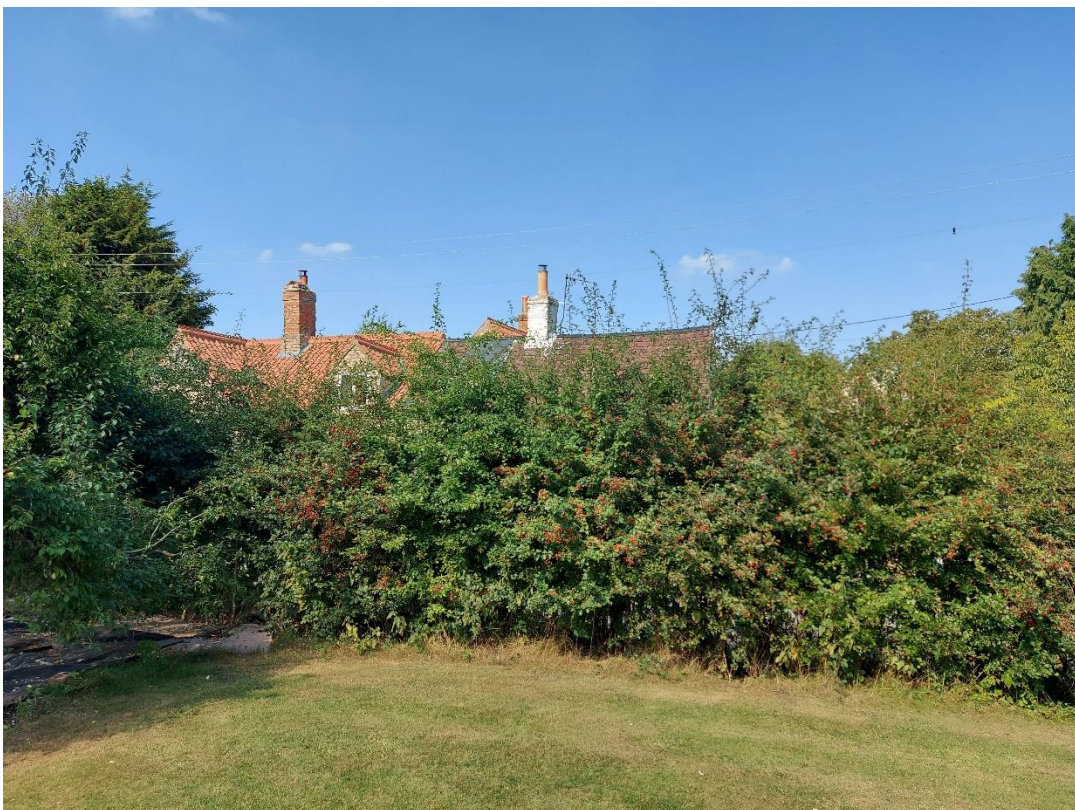
View towards Westons Cottage
