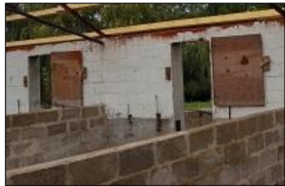
Figure 6: Pinned back wooden doors on eastern aspect.
