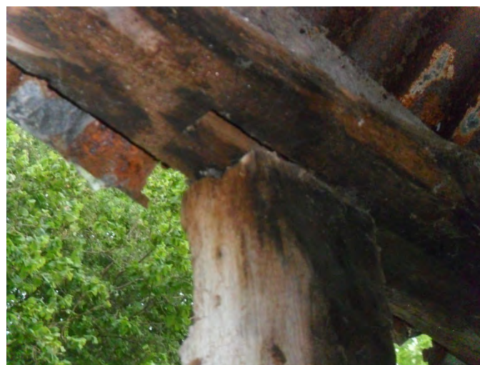
Open mortise/tenon joints
