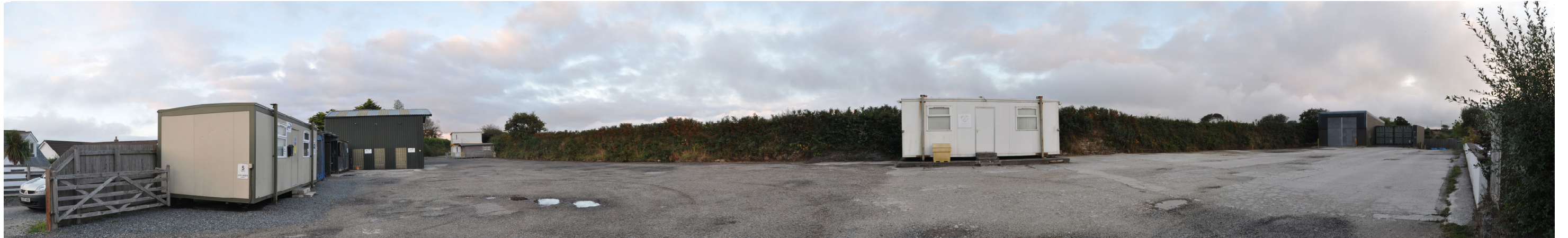
View of existing yard from site access point
