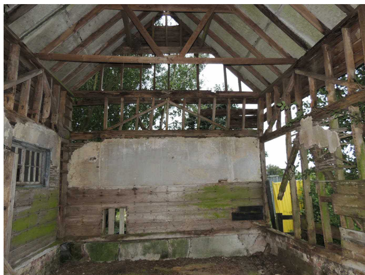
Photo 7: Looking NW at northern end of the barn
