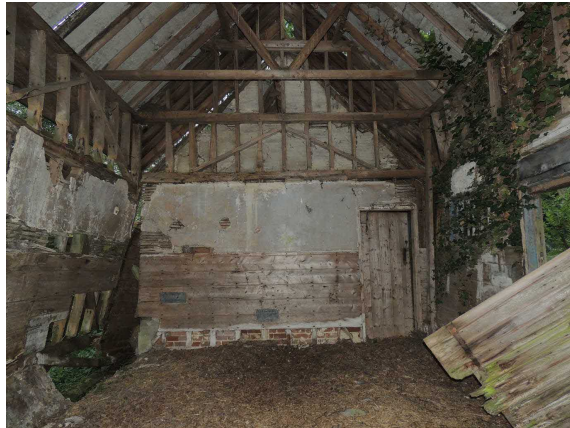
Photo 8: Looking SE at NW end of barn
