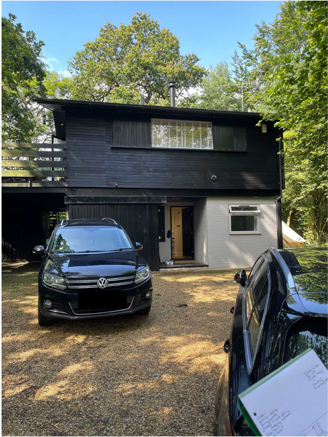
Front view showing the existing entrance and balcony to the side
