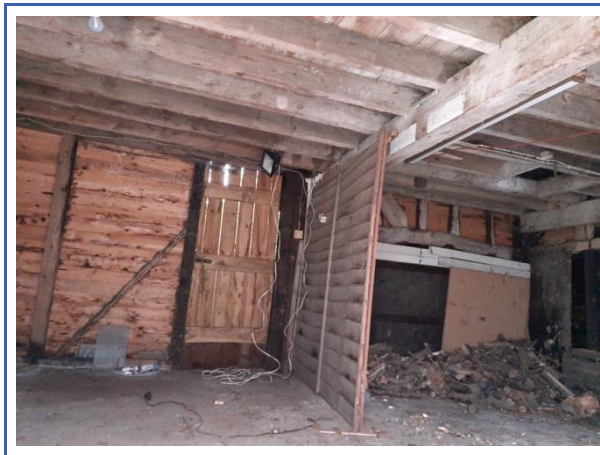
Internal view of the barn and log pile on site
