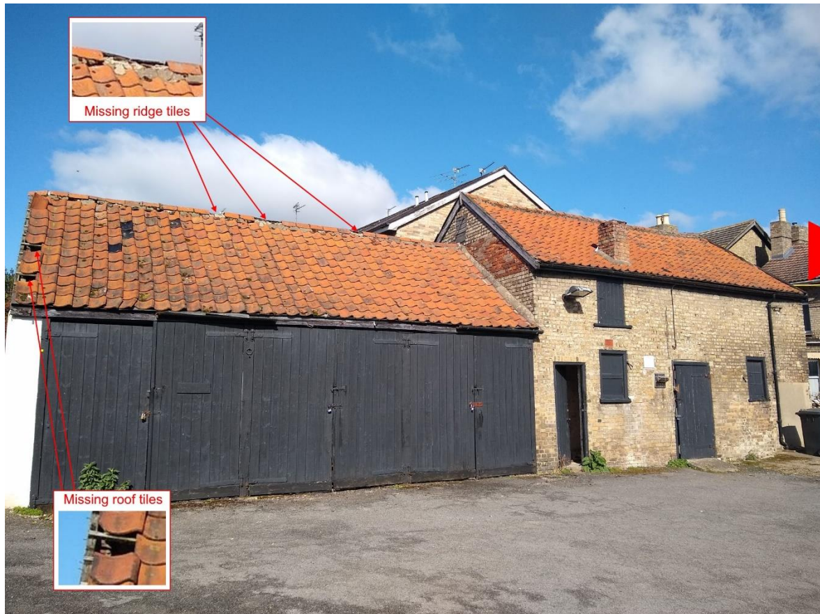
Image 4.3.2.1. Location of bat access points on the south-east elevation of the outbuilding.
