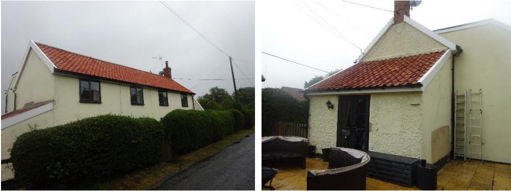
Existing front elevation photo (above left) side elevation (above right)
