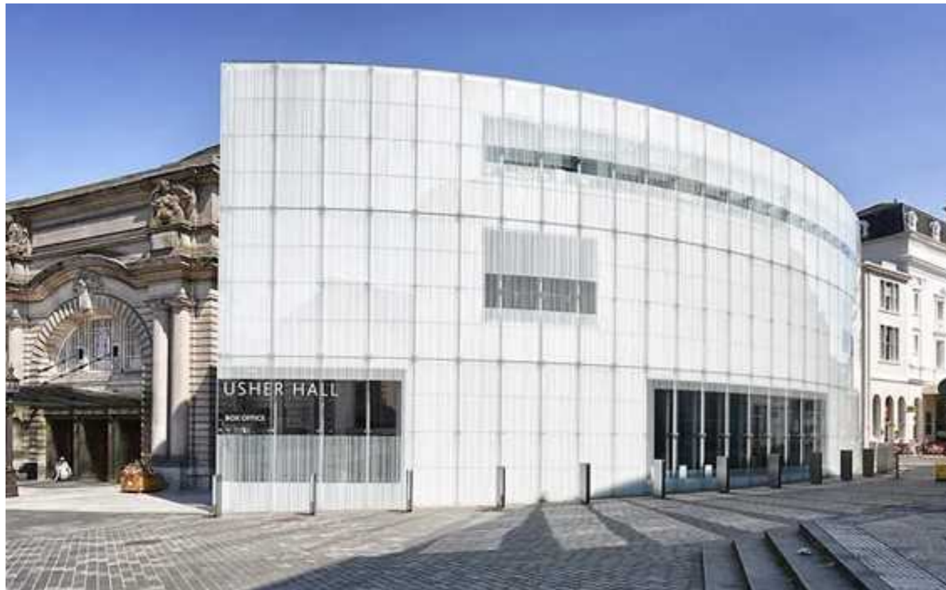
Usher Hall extension, Edinburgh, LDN Architects
