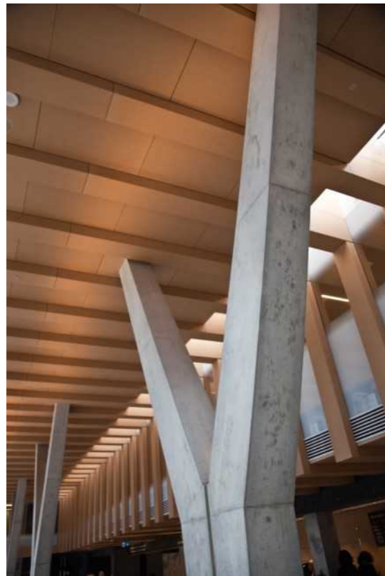
Example of a sculptural concrete column
