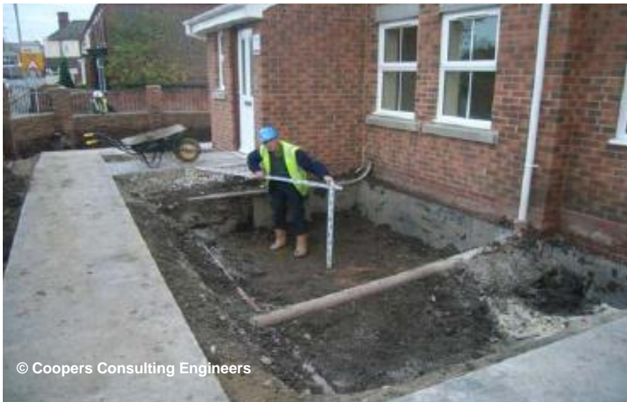
© Coopers Consulting Engineers
