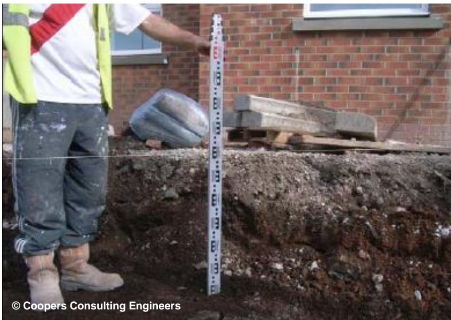
© Coopers Consulting Engineers
