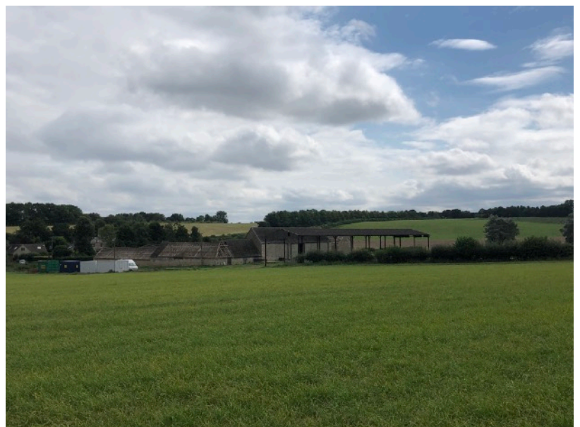
Fig. 1 Site looking west before commencement of works.
